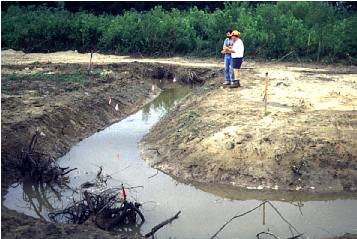
Stream Restoration Project showing new meander
