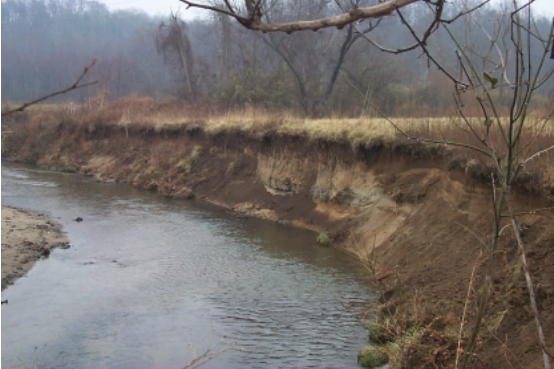
Brasstown Creek, showing bank instability and no buffer.
