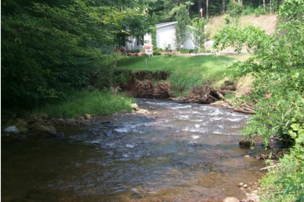
Shooting Creek, east of Hayesville, showing bank instability next to a residence.
