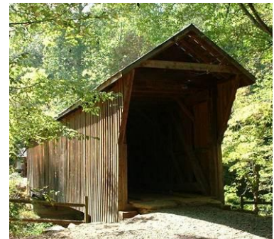
Figure 5. Bunker Hill Bridge over Lyle Creek.
