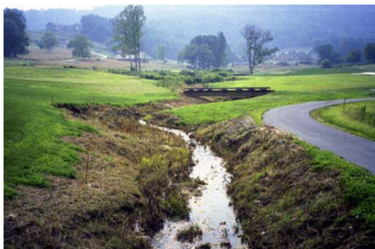
Stream restoration project on County Line Creek, Buncombe County
