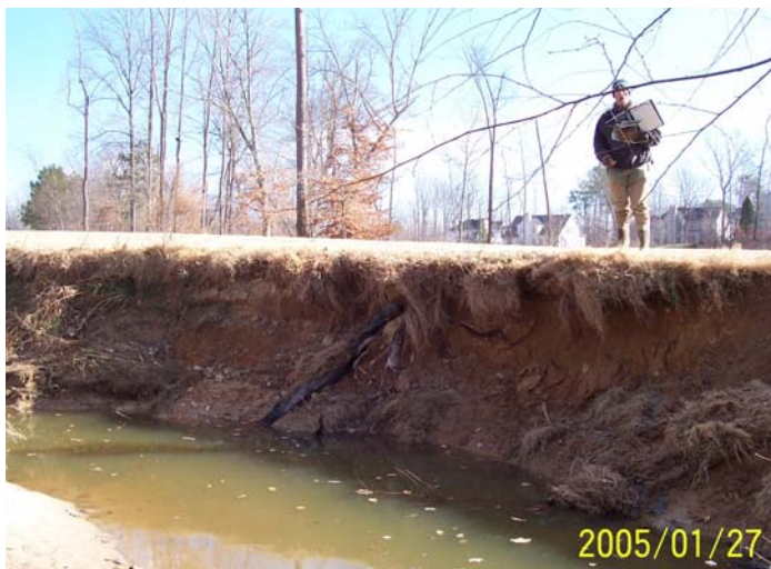
Severe Streambank Erosion in Little Lick
