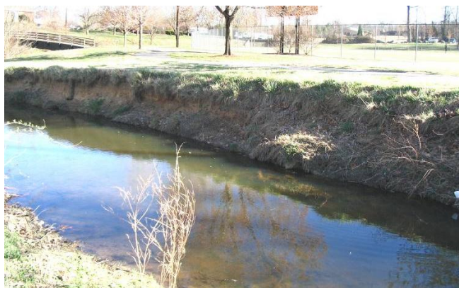
Figure 1. Streambank erosion at Burlington's City Park contributes to pollution in Little Alamance Creek. This site has been targeted for a stream restoration project.
