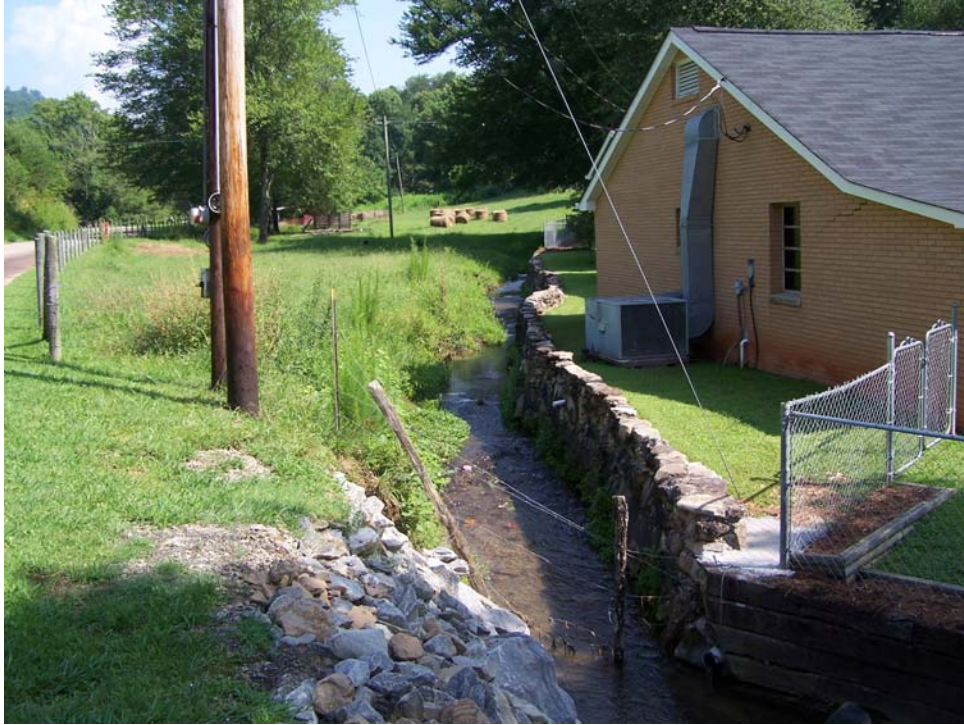
Site R-1. Moore Branch (shown on USGS maps as Fate Puett Cove Creek) at SR 1538. Upstream view from road culvert.
