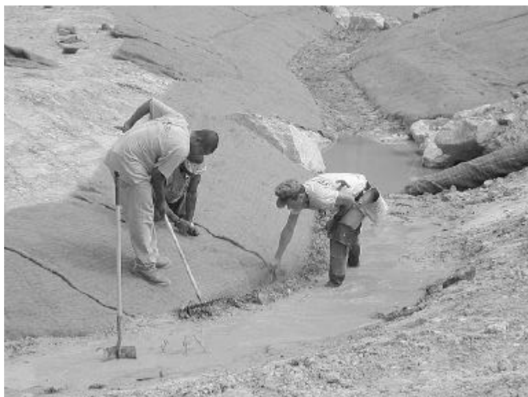
Men at work on stream restoration project
