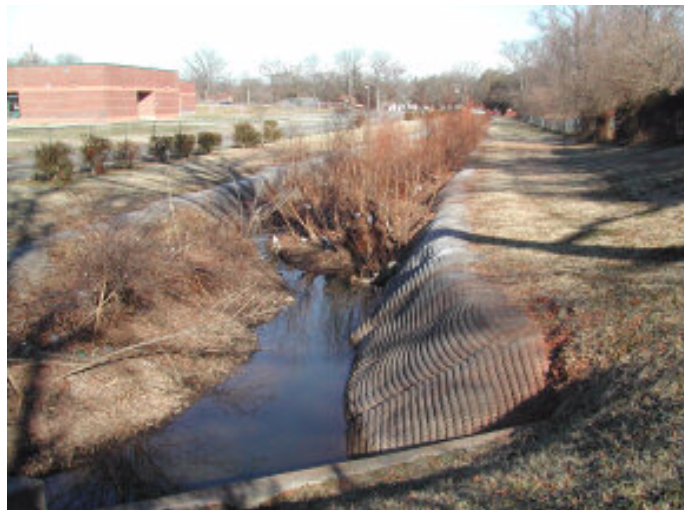
Goose Creek, Urban Restoration Project Durham County
