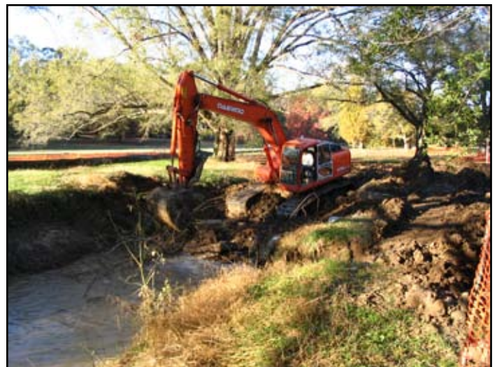
Returning the waterway to a more natural meander
